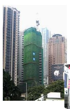
A few buildings that were being worked on had a complete wrapping of green screening material around them as a safety containment and protection for the workers.
